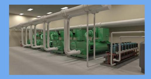
(4) 1,300 TON CENTRIFUGAL CHILLERS (4) 18,000 MBH COOLING TOWERS (1) 200 TON HEAT RECOVERY CHILLER DOMESTIC HOT WATER & CHILLED WATER PROVIDES 44°F TO AHUS
